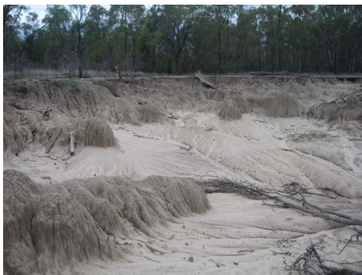
PLATE 5.1 SIGNIFICANT EROSION ADJACENT TO KOGAN CREEK.
