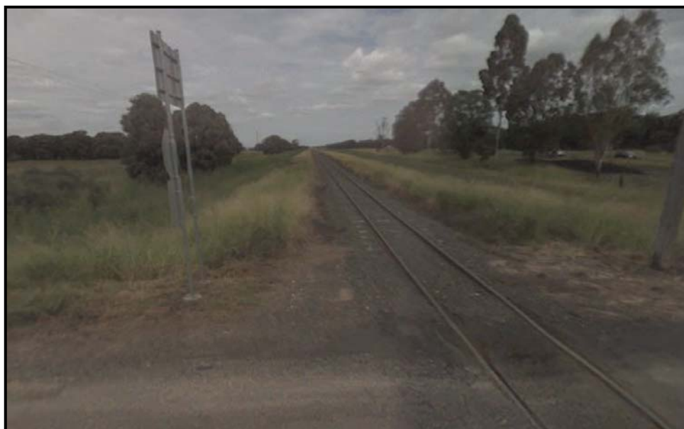
FIGURE 16.5 RAIL LINE NEAR THE STUDY AREA
