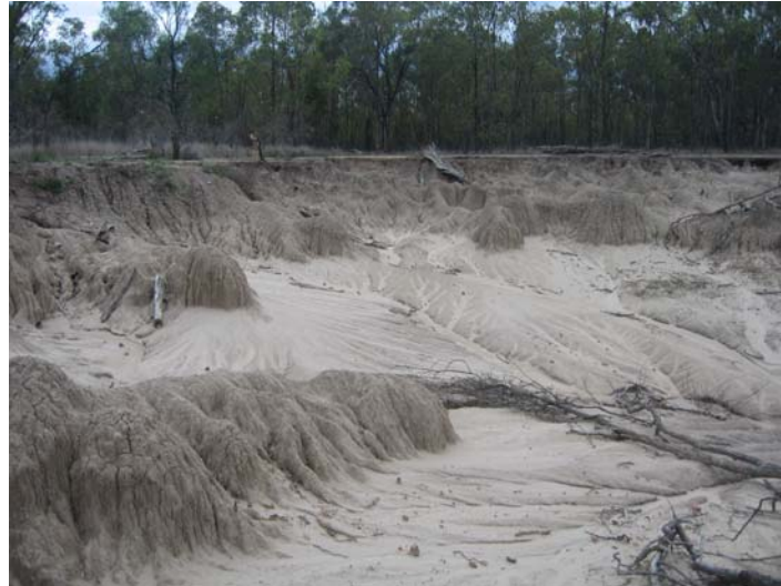
PLATE 5.1 SIGNIFICANT EROSION ADJACENT TO KOGAN CREEK.
